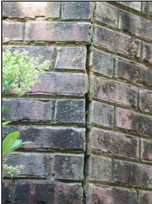
2.3 Picture 2 brick opening
