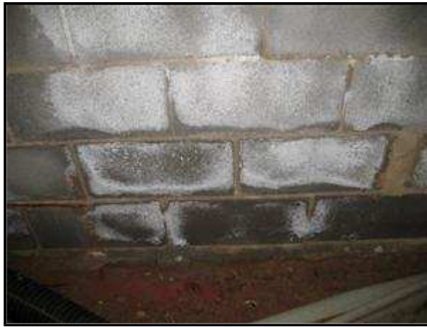
5.0 Picture 1 Efflorescence
