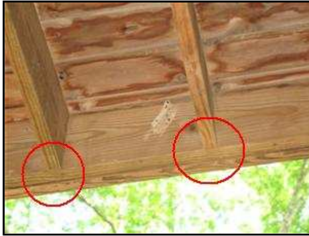
2.3 Picture 1 Joist Support
