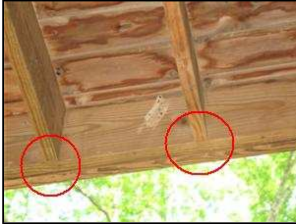
Item 4 - Picture 1 Joist Support
